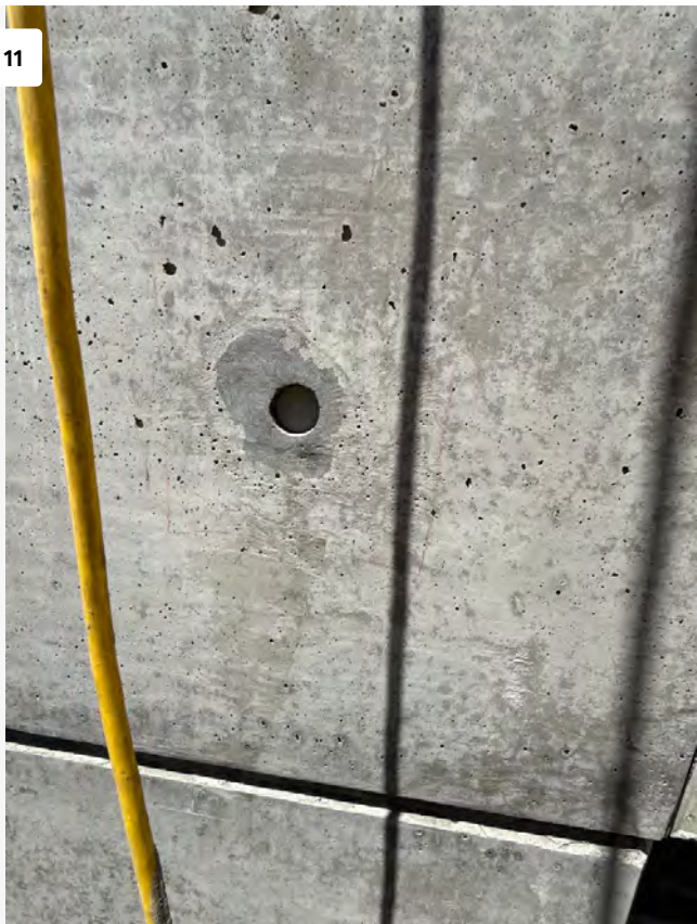
View of Repaired Spalling.
