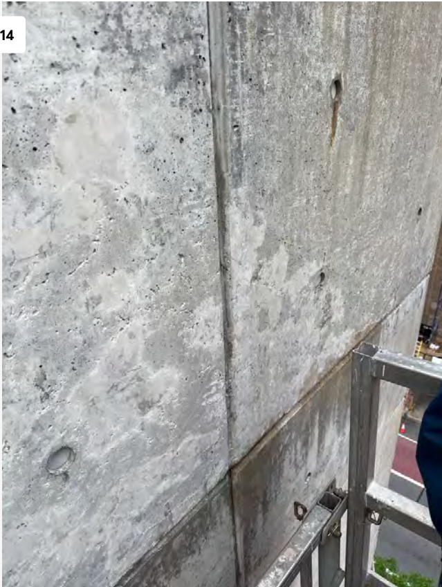
View of Area to be Grinded Down.
