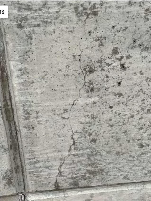
View of Crack to be Repaired
