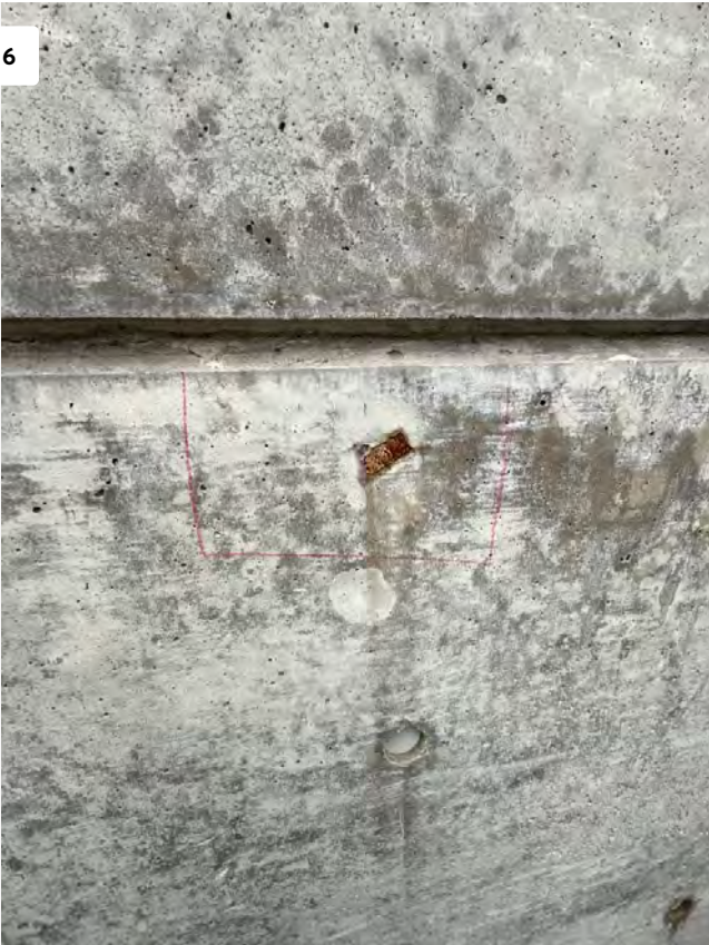
View of Wood Embedded into Facade. To Be Removed
