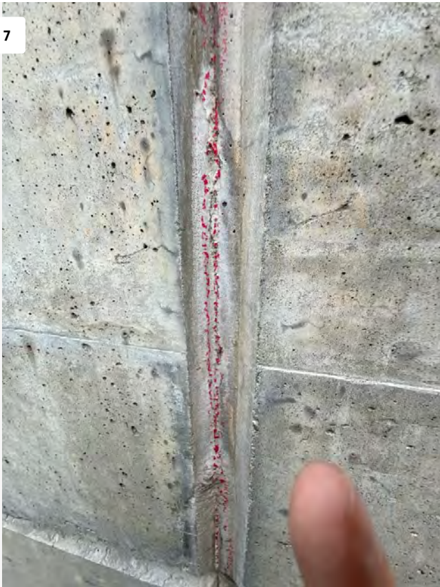
View of Crack in Recess of Parapet to be Repaired
