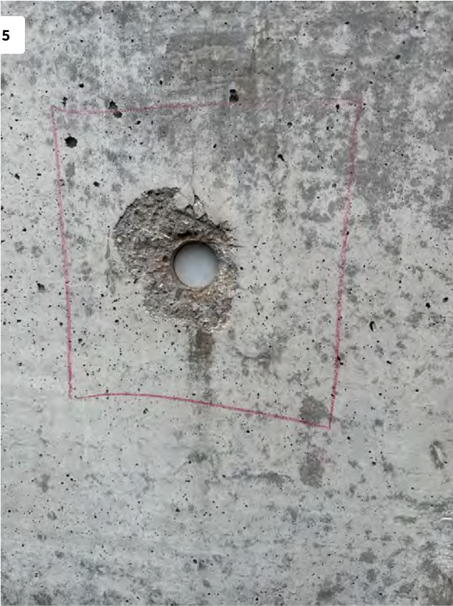
View of Spalled Concrete Around Port Hole
