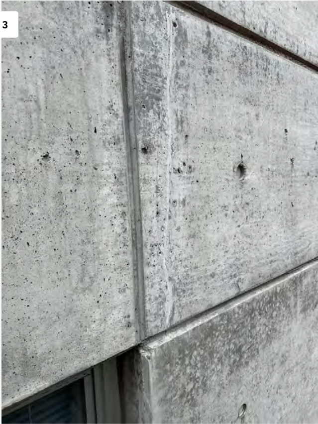
View of Completed Crack Repair
