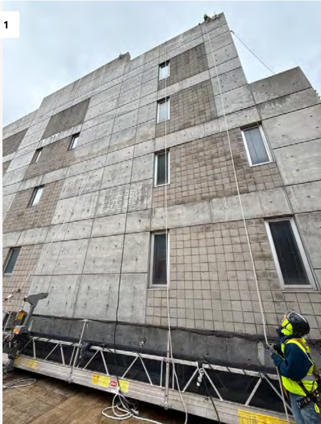
View of Scaffold Setup at West Elevation
