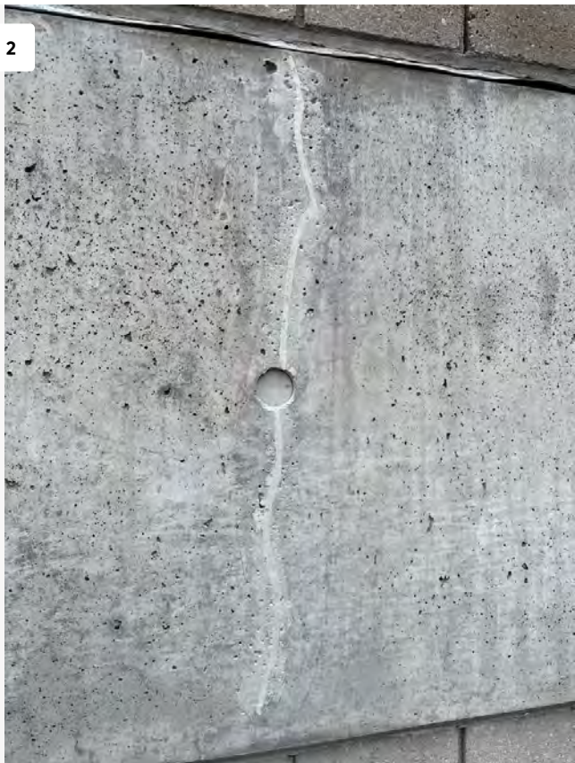
View of Completed Crack Repair
