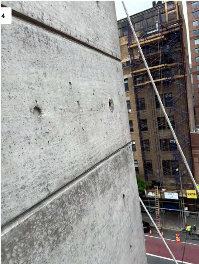
View of Spalled Concrete Around Port Hole
