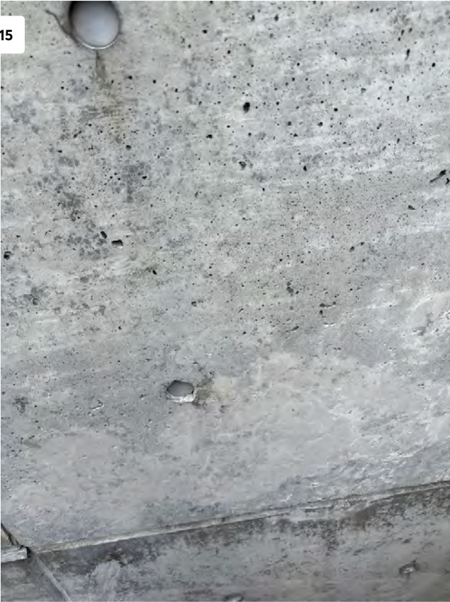
View of Area to be Grinded Down.
