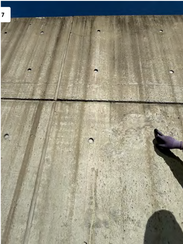
Crack Repair in Progress
