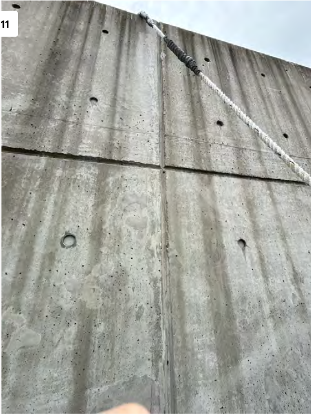
Crack Repair at Bulkhead
