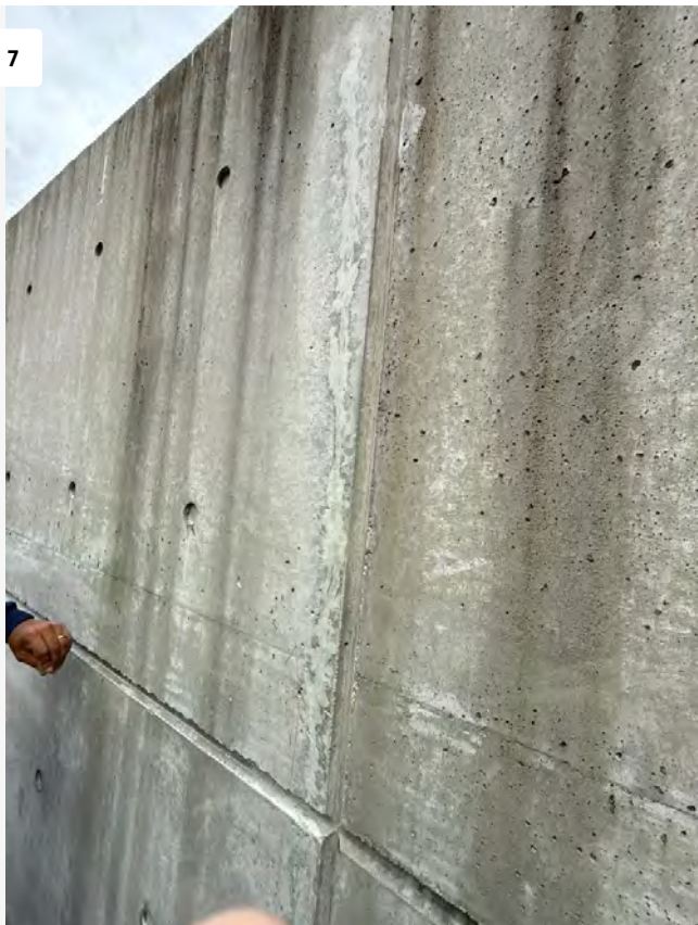
Crack Repair at Bulkhead
