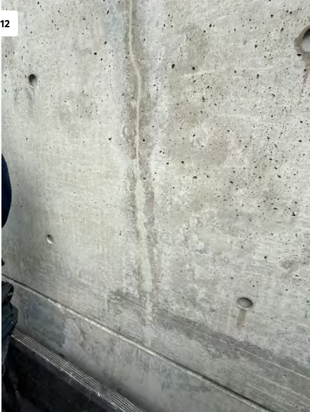
Crack Repair at Bulkhead
