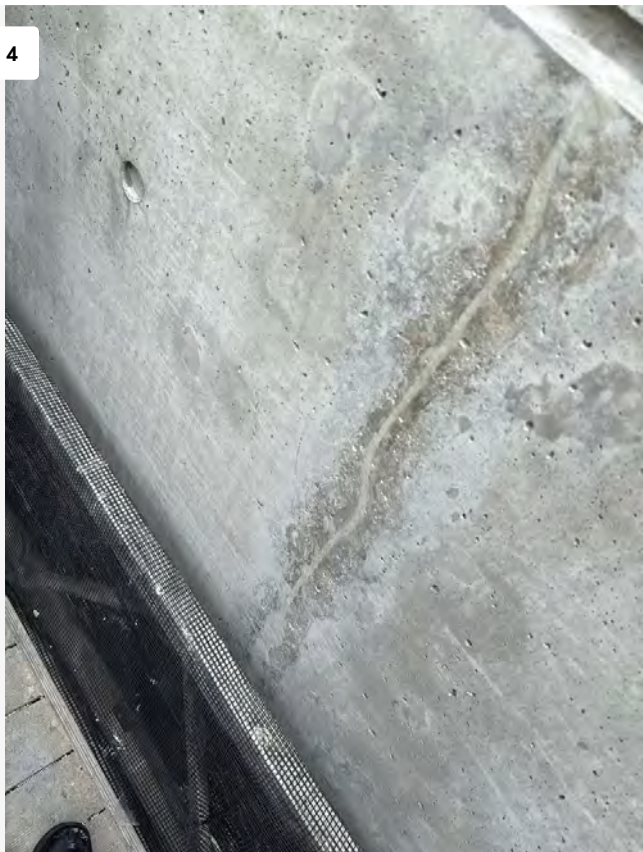
Crack Repair at Bulkhead
