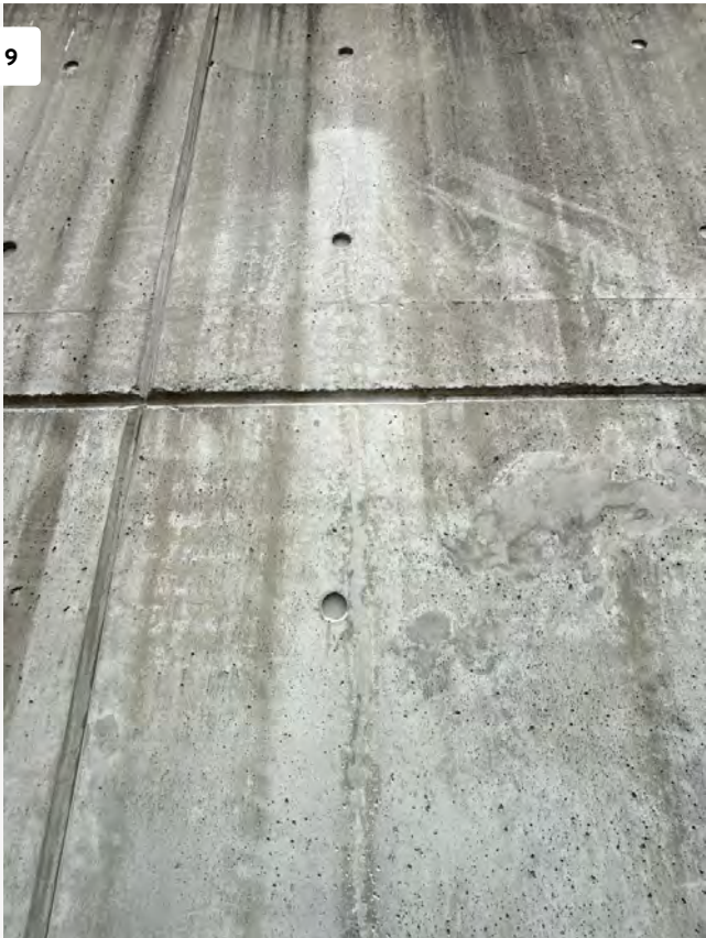
Crack Repair at Bulkhead
