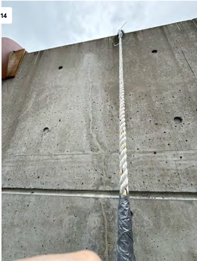
Crack Repair at Bulkhead
