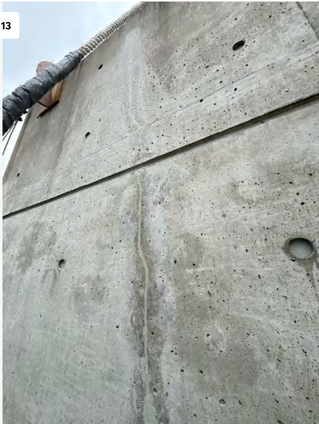
Crack Repair at Bulkhead
