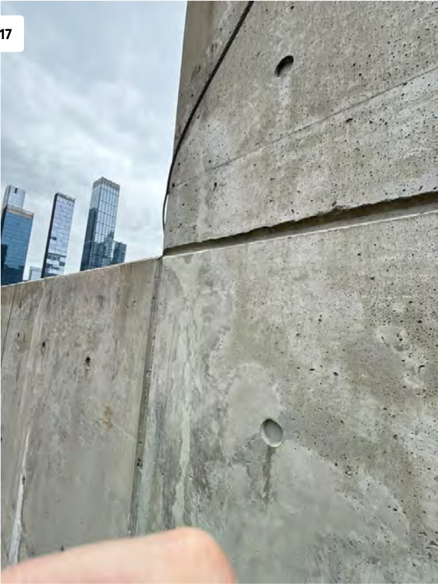
Crack Repair at Bulkhead
