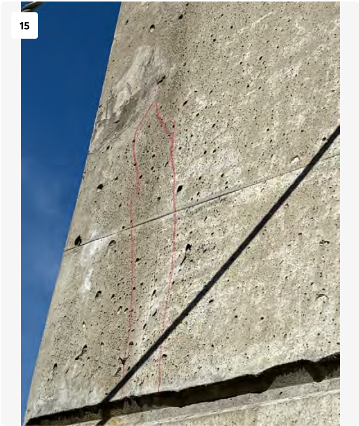
Crack Repair in Progress
