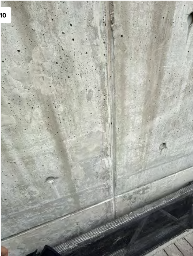
Crack Repair at Bulkhead
