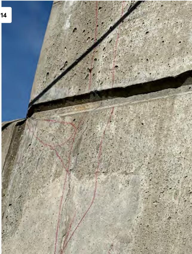
Crack Repair in Progress
