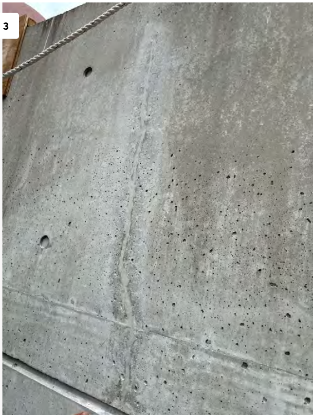
Crack Repair at Bulkhead
