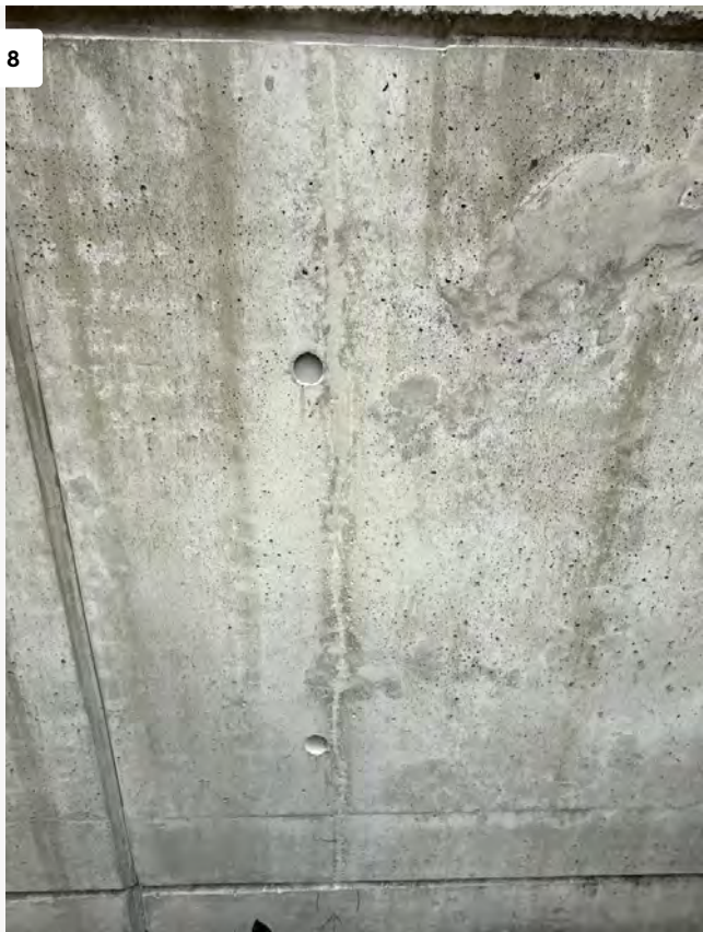
Crack Repair at Bulkhead
