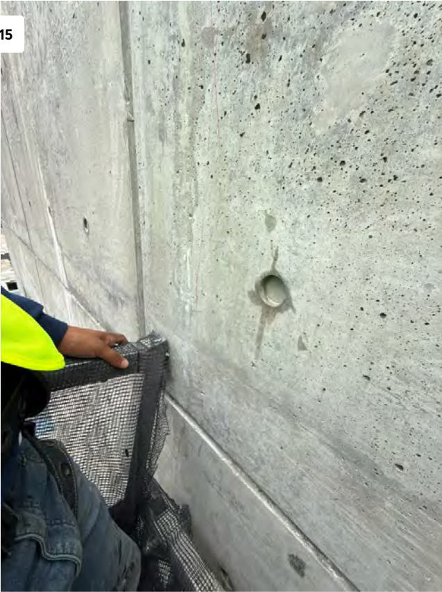
Crack Repair at Bulkhead
