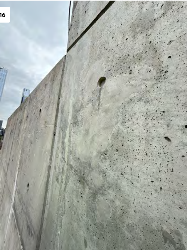
Crack Repair at Bulkhead
