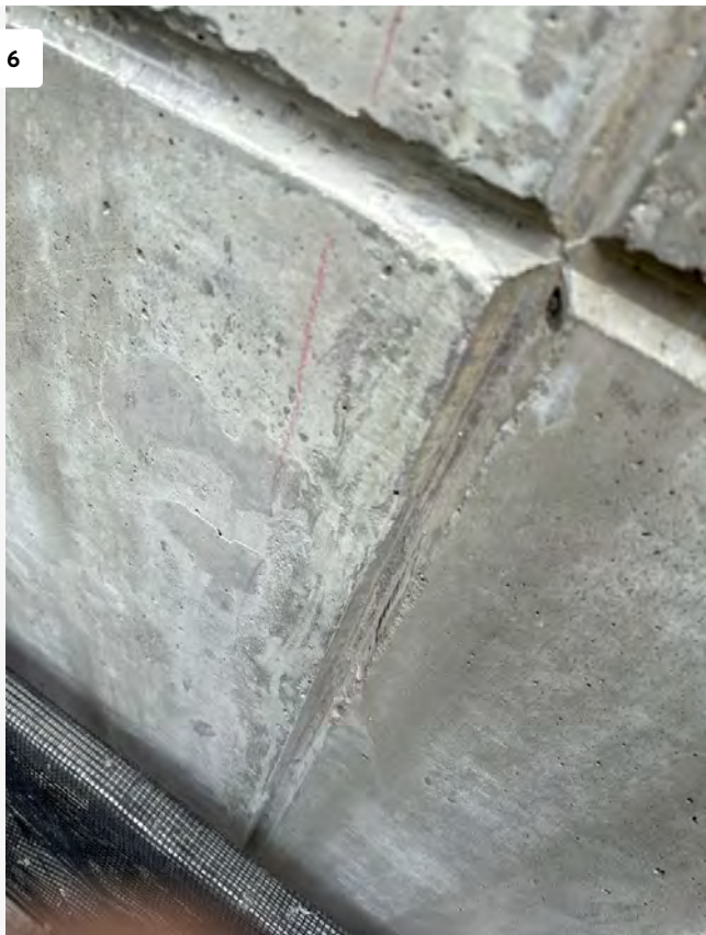
Crack Repair at Bulkhead
