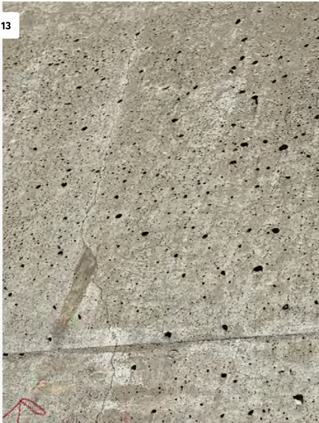
Crack Repair in Progress
