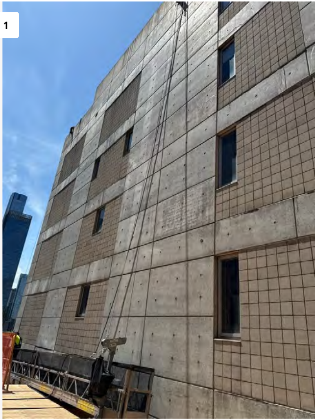
View of Scaffold Setup at East Elevation
