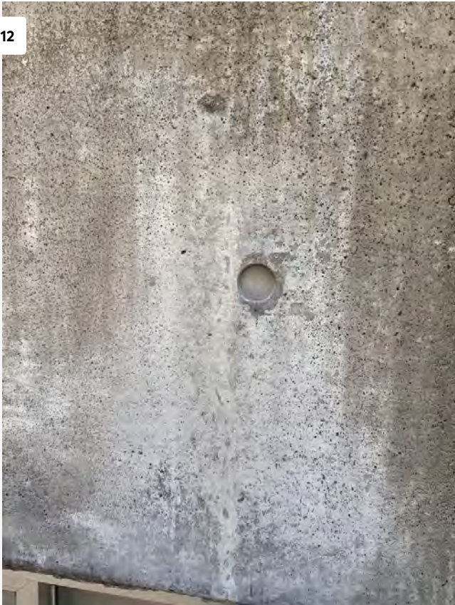
View of Completed and Cleaned Crack Repair at North Elevation
