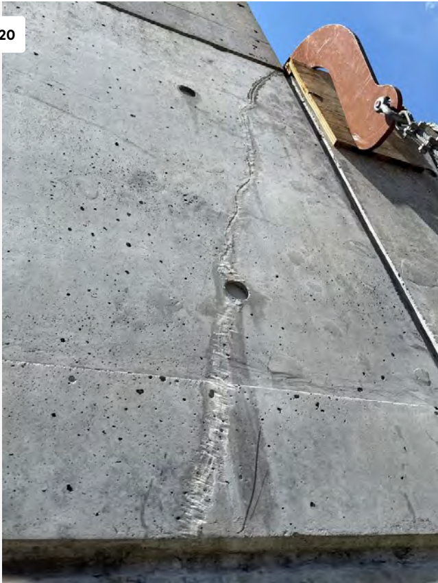
View of Completed Crack Repair at East Elevation. Clean up of Area Pending
