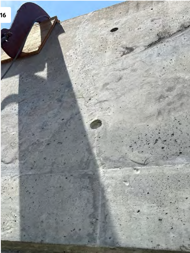
View of Completed Crack Repair at East Elevation
