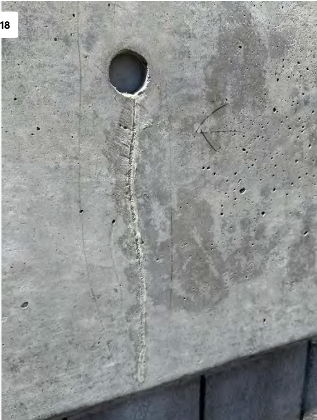
View of Crack Repair at East Elevation. Further Grinding Required
