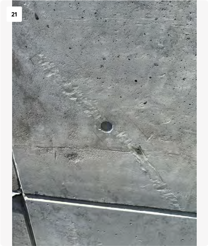
View of Completed Crack Repair at East Elevation
