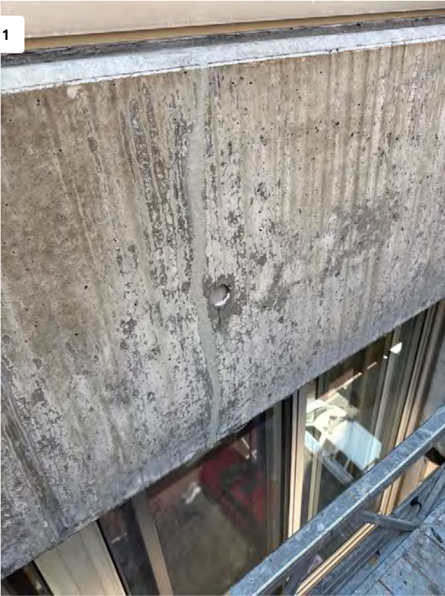
Crack Repair at North Elevation
