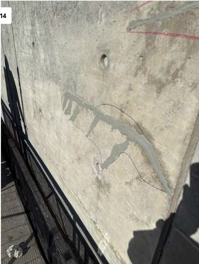
Crack Repaired at East Elevation
