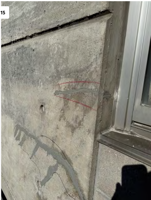
Crack Repaired at East Elevation
