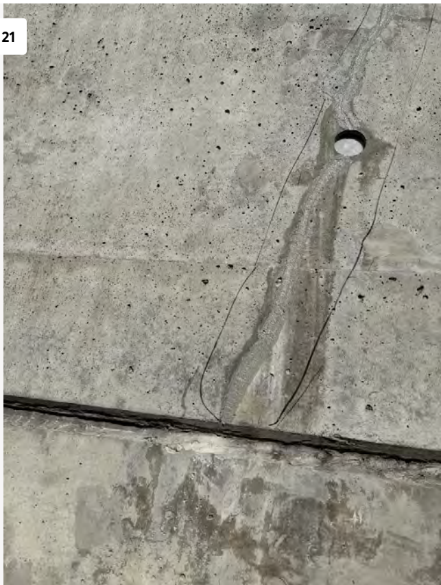
Crack Repaired at East Elevation
