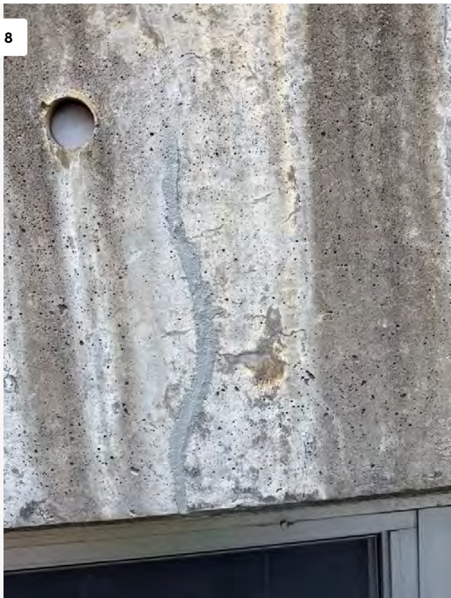
Crack Repaired at North Elevation
