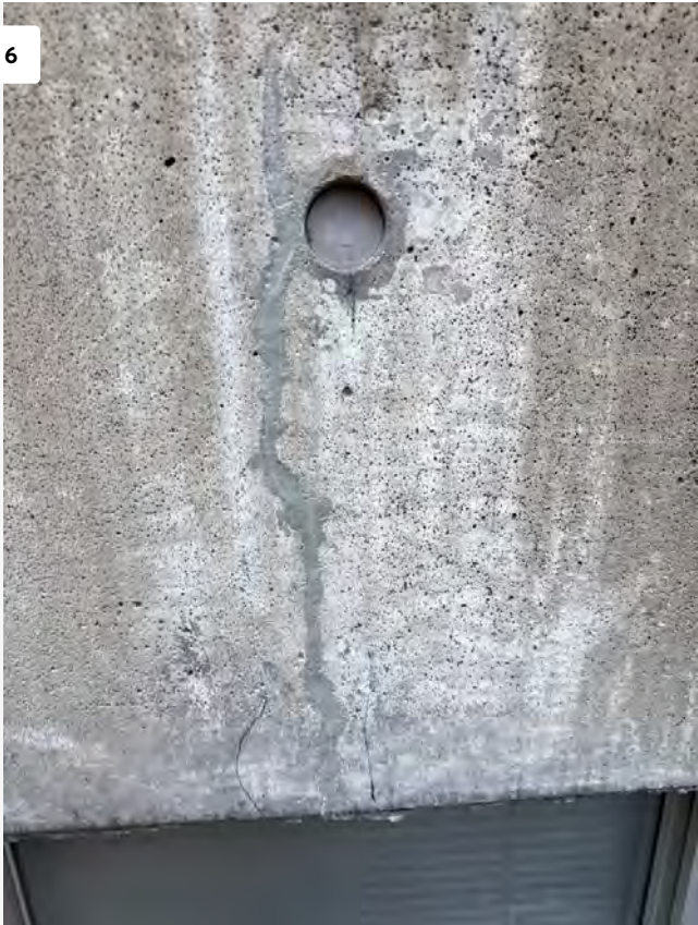
Crack Repaired at North Elevation
