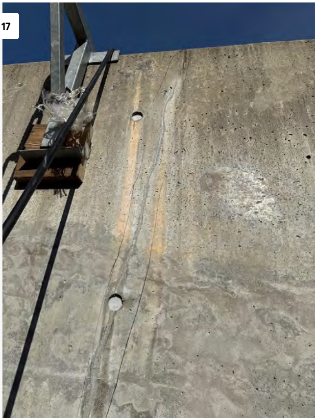
Crack Repaired at East Elevation
