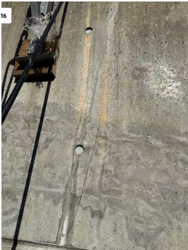
Crack Repaired at East Elevation
