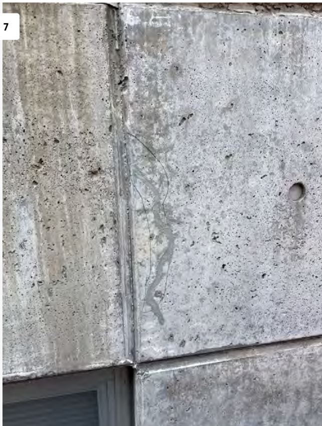
Crack Repaired at North Elevation
