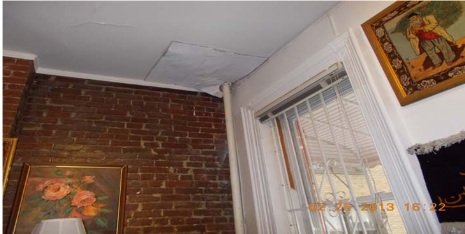
REAR 1 ST FLOOR – WATER SEEPAGE ON CEILING
