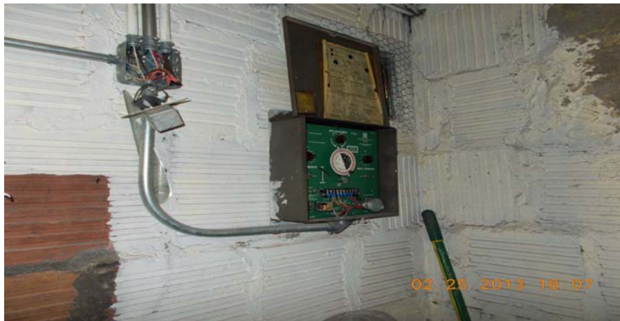
THERMOSTAT INSIDE BOILER ROOM TO CONTROL HEATING TEMPERATURE
