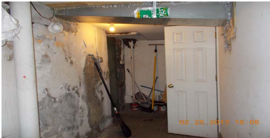
FRONT BASEMENT ENTRANCE AREA – FOUNDATION WALL SPALLING
