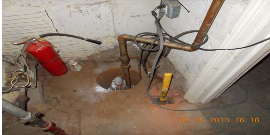
SUMP PIT & PUMP INSIDE BOILER ROOM
