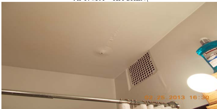
APT. #3A - BATHROOM CEILING - PAST LEAKS
