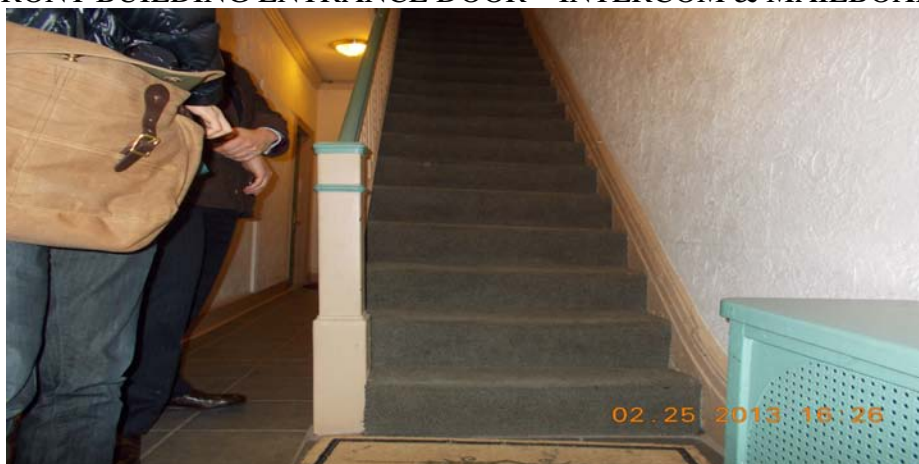
FRONT STAIR TO APARTMENTS SLIGHTLY SAGGING
