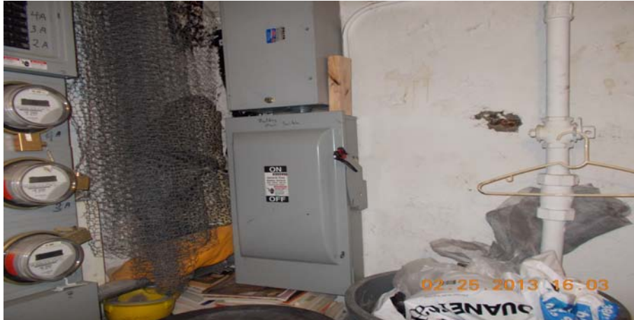
MAIN ELECTRIC SHUTOFF PANEL FOR BUILDING
