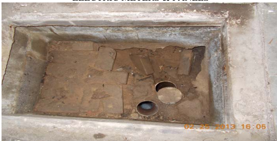
HOUSE TRAP & SEWER CLEANOUT – NEEDS COVERING CLEANOUT
