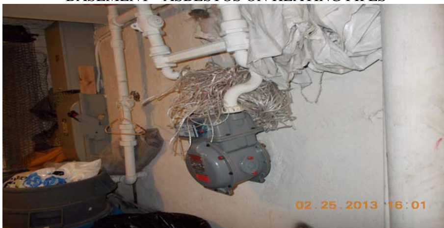
GAS METER FOR BUILDING - HEATING & HOT WATER
