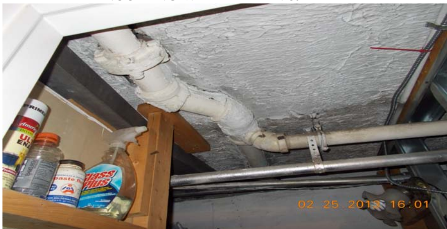
BASEMENT - ASBESTOS ON HEATING PIPES
