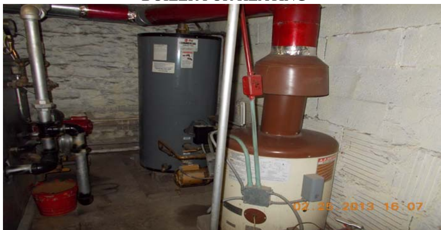
HOT WATER BOILER & STORAGE TANK
