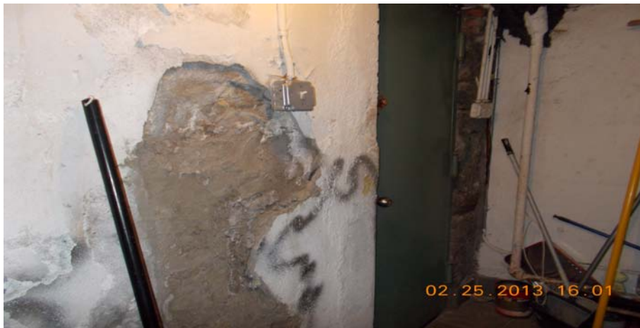
BASEMENT FRONT ENTRANCE DOOR – SPALLING FOUNDATION WALL
