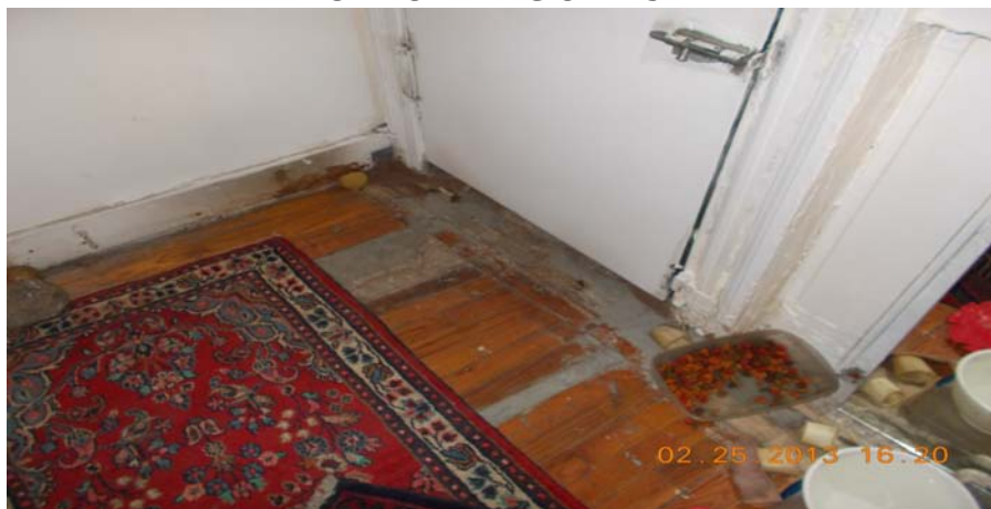
REAR BASEMENT – ROTTED & SOFT HARDWOOD FLOORING IN FRONT OF DOOR
