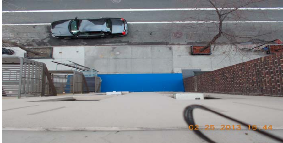
FRONT OF BUILDING LOOKING DOWN
