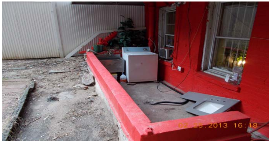
REAR OF BUILDING & BASEMENT
