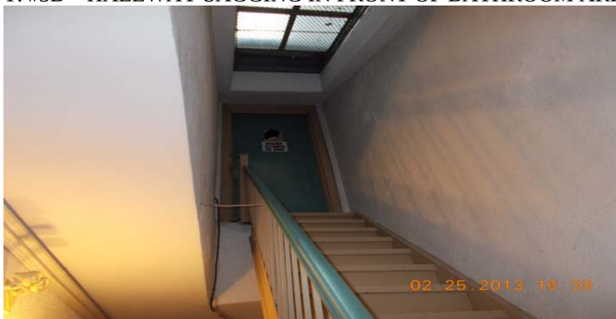
STAIR TO ROOF
