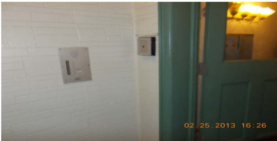
FRONT BUILDING ENTRANCE DOOR – INTERCOM & MAILBOXES
