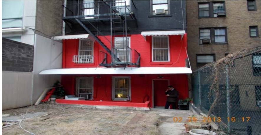
REAR OF BUILDING & REAR YARD
