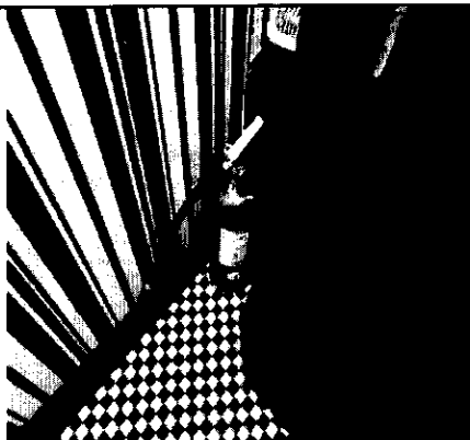
fire extinguisher-no tag and unmounted
