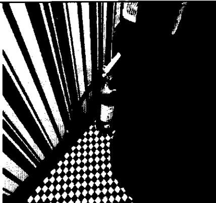
fire extinguisher-no tag and unmounted
