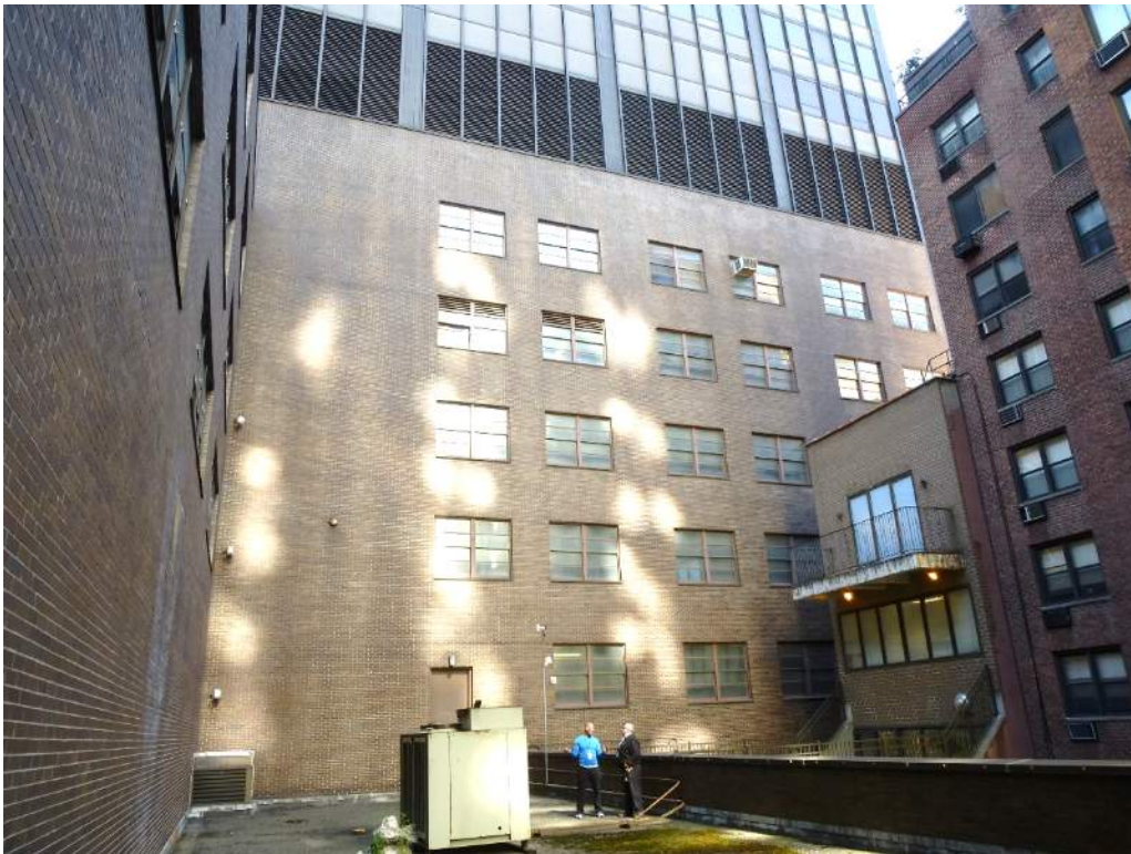
Elevation Photo No. 6 - Overall view of lower West Elevation.
