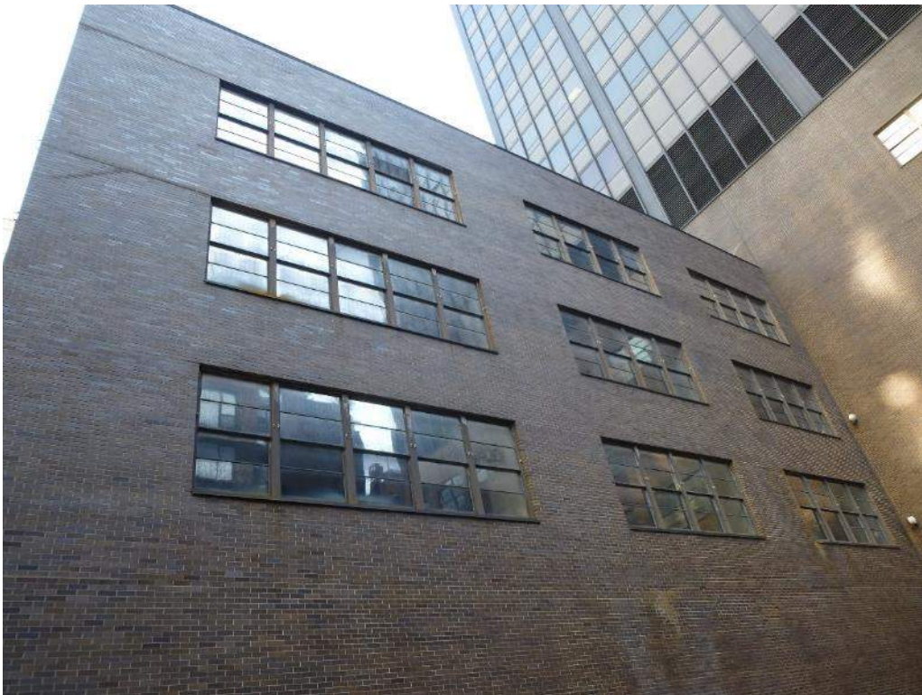
Elevation Photo No. 7 - Overall view of recessed South Elevation (school building).
