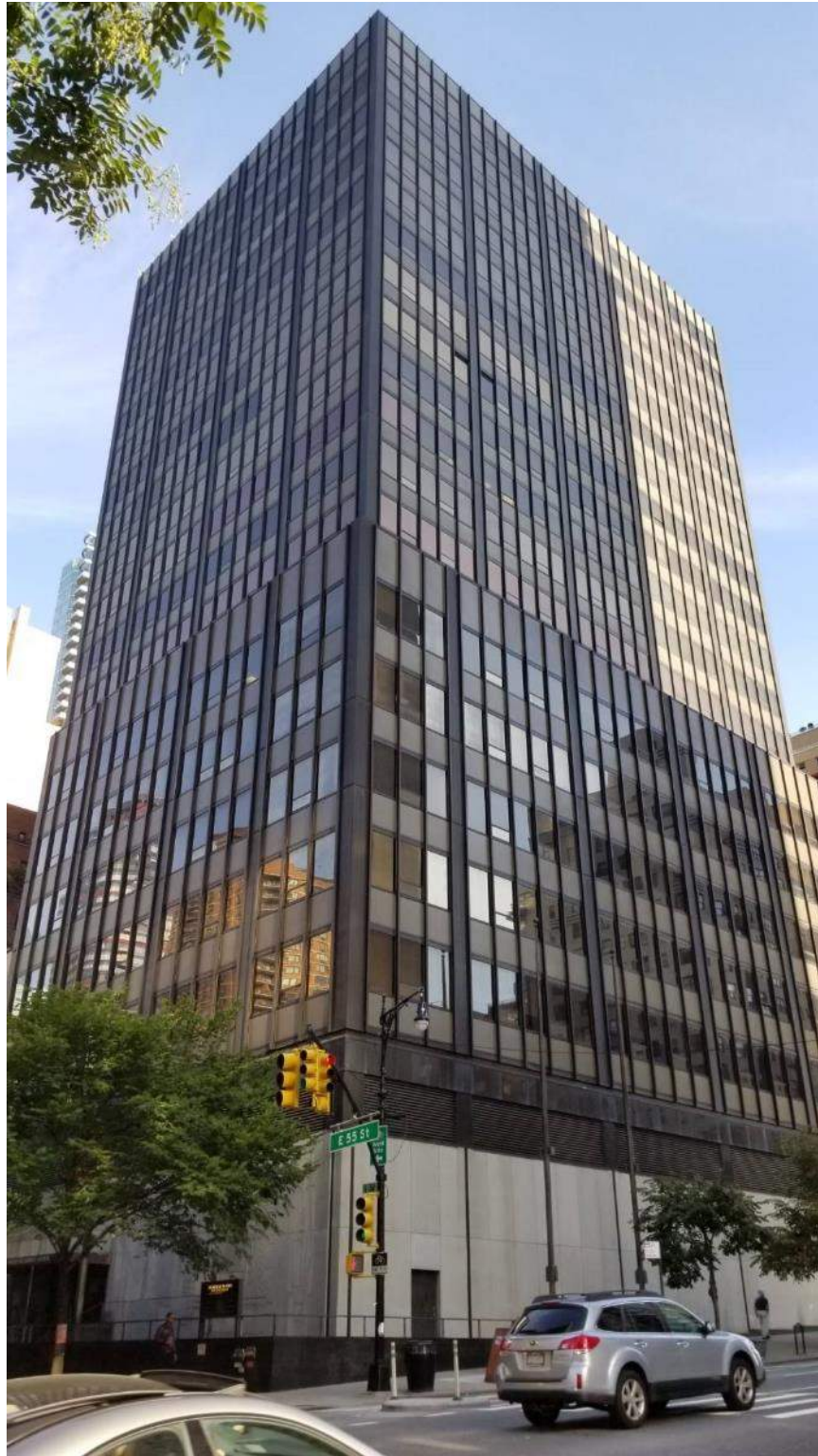
Elevation Photo No. 2 - Overall view of South and East Elevations from 1 st Avenue.
