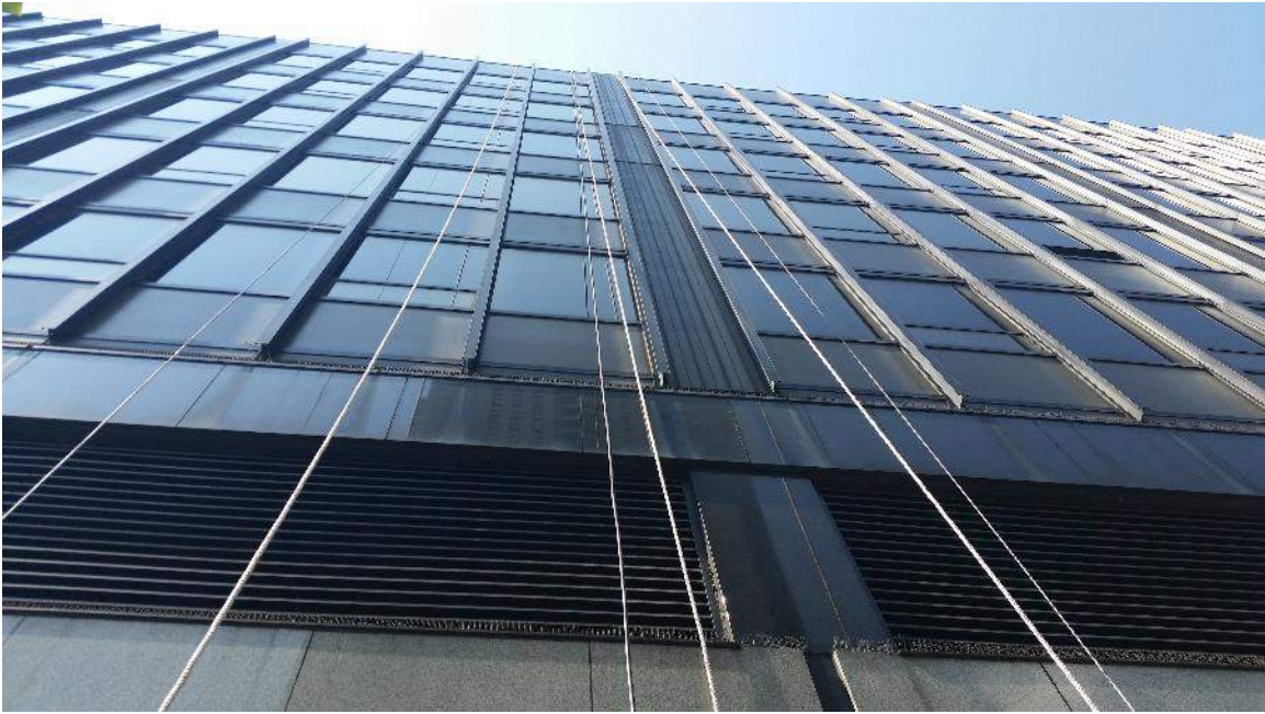
Detail Photo No. 1 - Overall view of East Elevation from 1 st Avenue.
