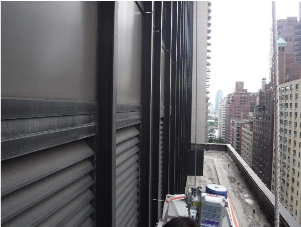
Detail Photo No. 15 - Overall view of South Elevation, curtain wall detailing.
