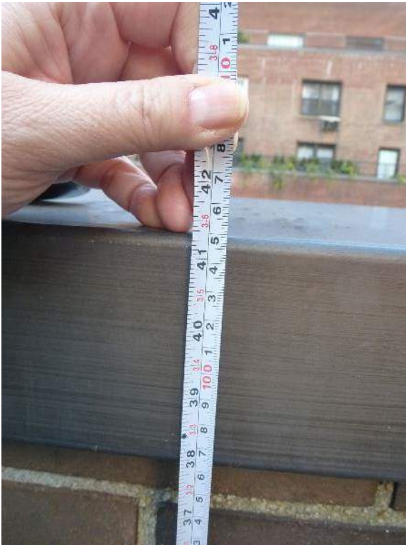
Detail Photo No. 38 – 7 th Floor Setback Roof - parapet height at 41½”.
