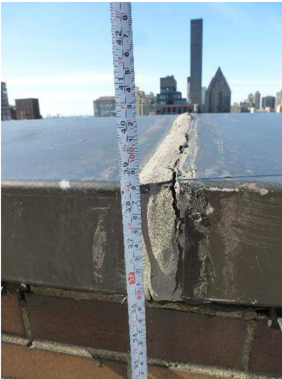
Detail Photo No. 33 – Main Roof – parapet height at 38½”.
