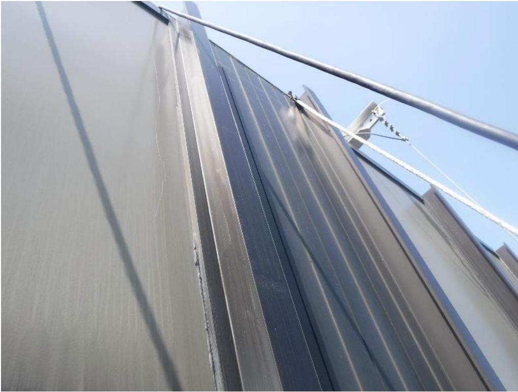
Detail Photo No. 3 - Overall view of East Elevation parapet exterior at top of building.
