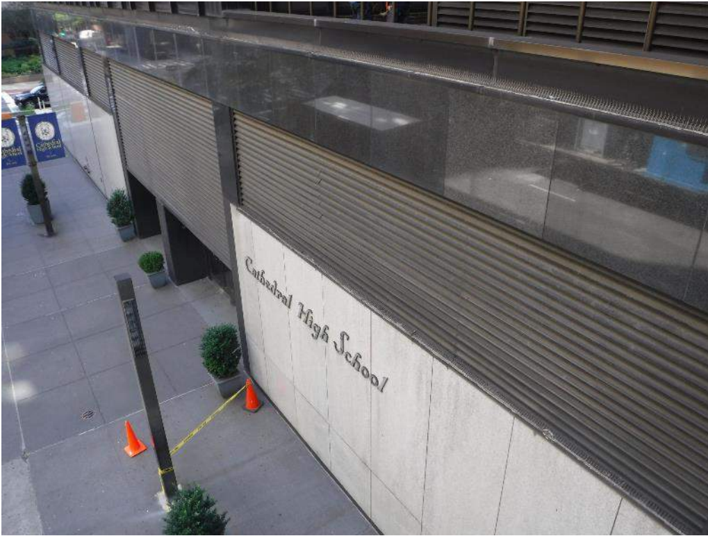
Detail Photo No. 13 - Overall view of North Elevation, lower floors.
