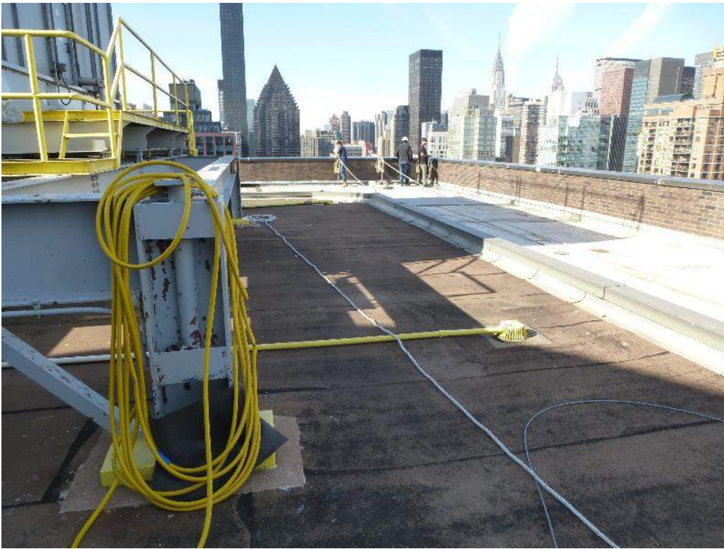
Detail Photo No. 33 – Main Roof looking north.
