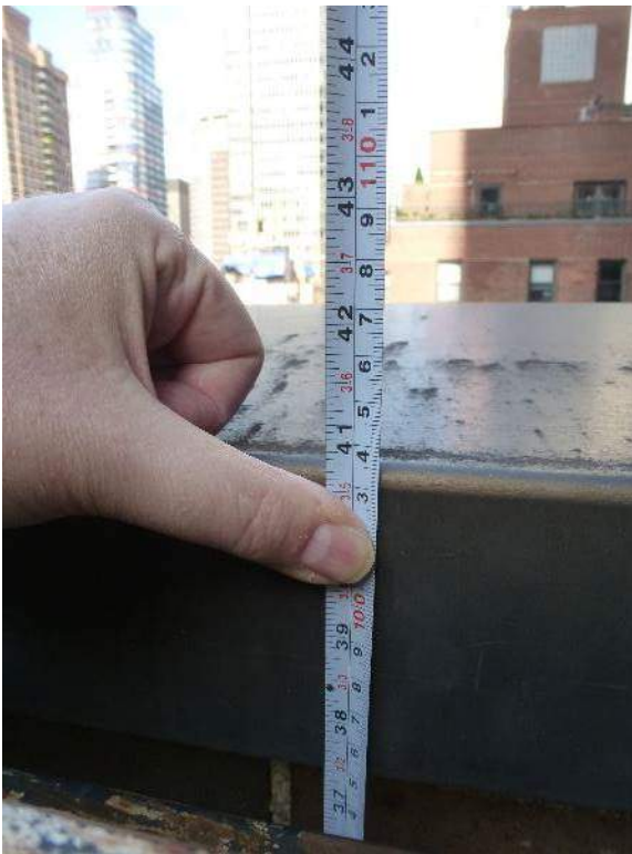
Detail Photo No. 36 – 8 th Floor Setback Roof - parapet height at 41".
