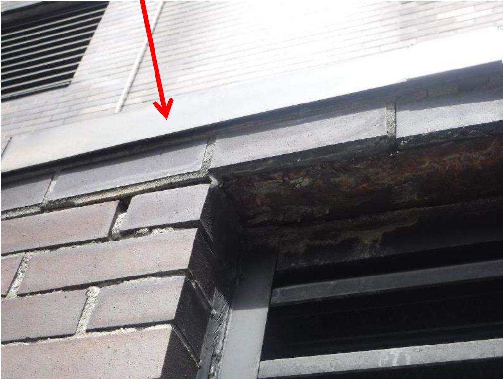
Detail Photo No. 20 – Overall view of South Elevation, masonry façade at Loading Dock entry – note open joints.
