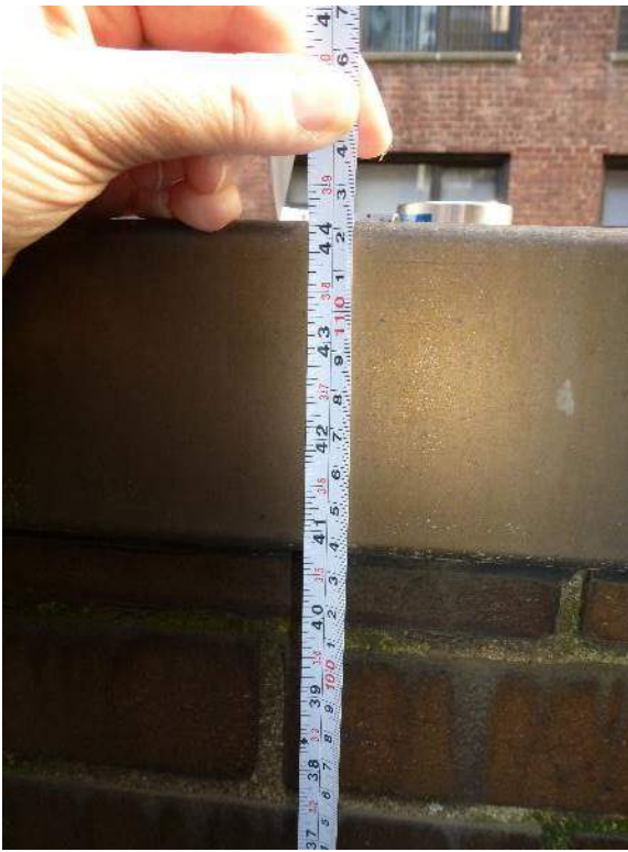
Detail Photo No. 40 – 3 rd Floor Setback Roof - parapet height at 44".
