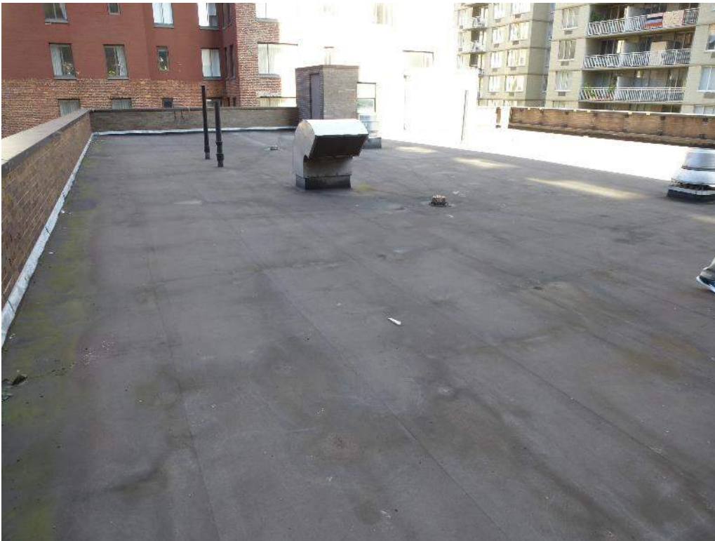
Detail Photo No. 37 – 7 th Floor Setback Roof looking west.
