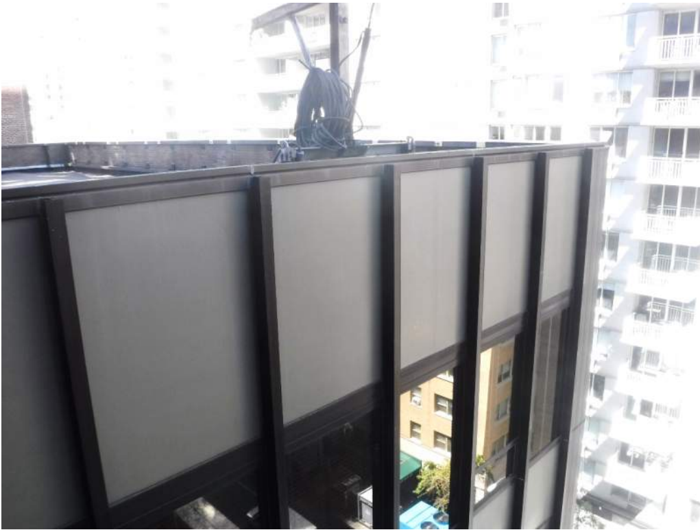
Detail Photo No. 11 - Overall view of North Elevation parapet exterior at 7 th Floor Setback Roof.
