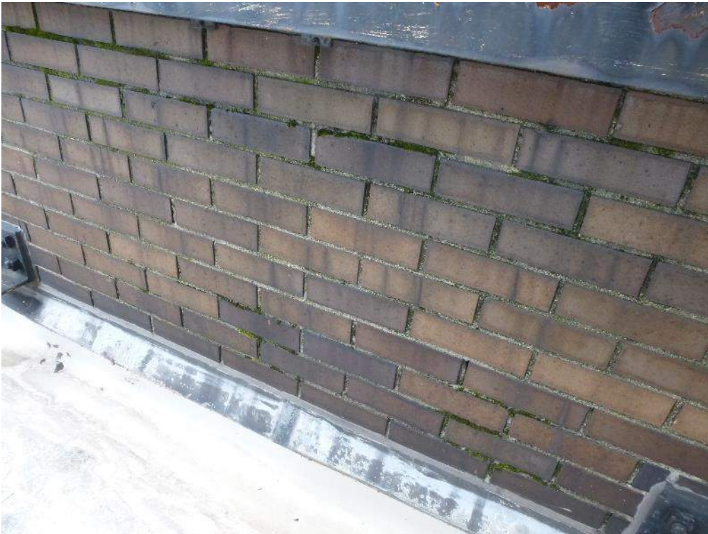
Detail Photo No. 42 – 8 th Floor Setback Roof parapet – deteriorated mortar joints..
