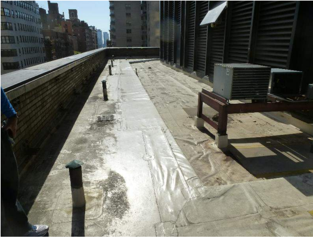
Detail Photo No. 35 – 8 th Floor Setback Roof looking east.
