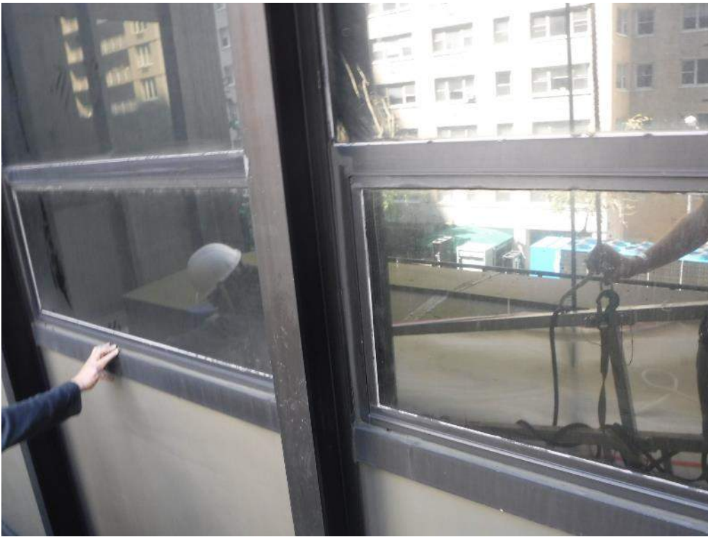
Detail Photo No. 9 - Overall view of North Elevation curtain wall detailing.
