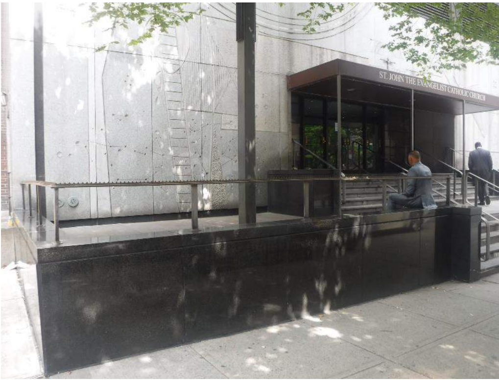
Detail Photo No. 21 - Overall view of South Elevation, granite façade at Church entry.
