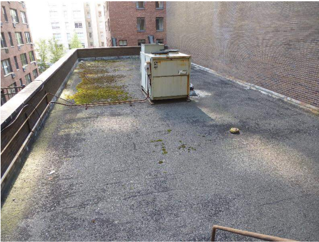
Detail Photo No. 39 – 3 rd Floor Setback Roof looking west.
