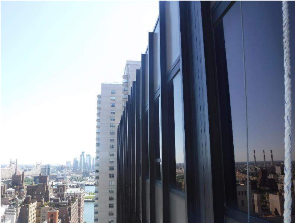
Detail Photo No. 7 - Overall view of North Elevation parapet exterior at top of building.
