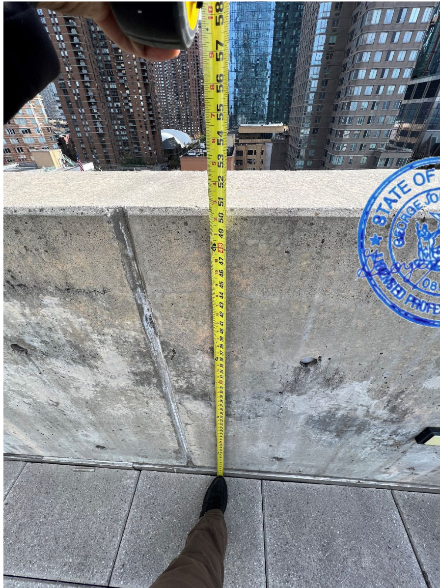
Picture 1 – Interior Parapet wall – Solid concrete wall with rebars. Approximately 50 inches in height. Typical Conditions
