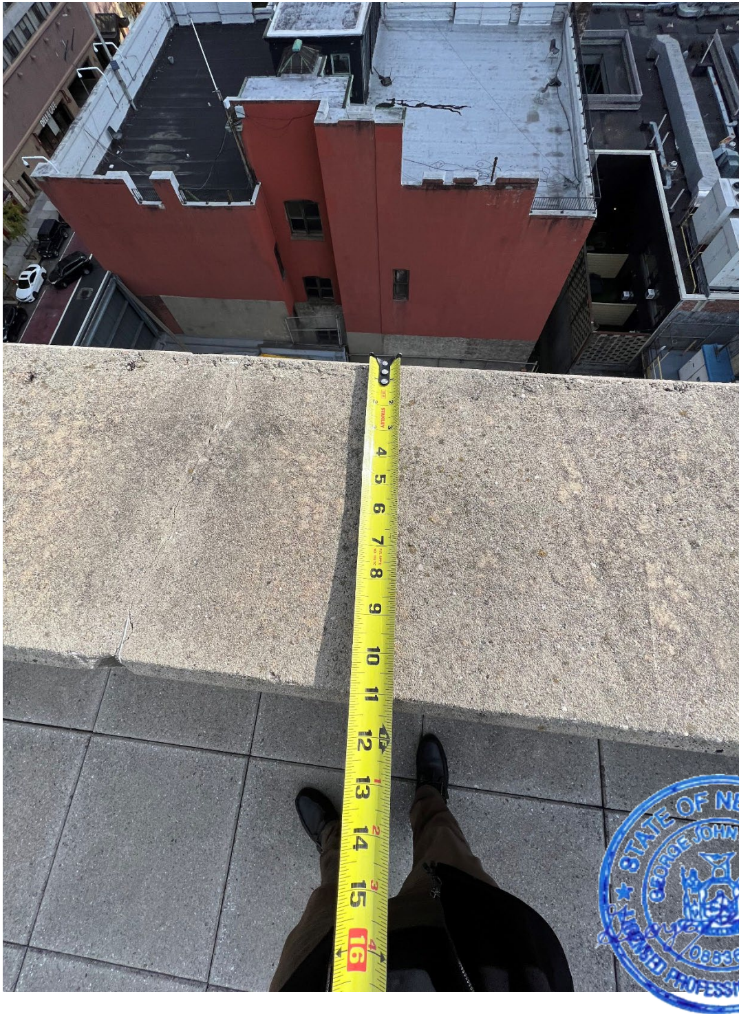
Picture 2 – Parapet wall – Solid concrete wall with rebar. Approximately 11 inches in width – Typical Conditions.
