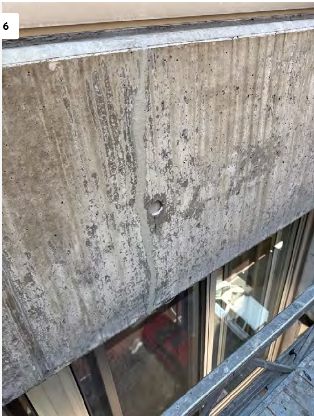
Typical View of Repaired Cracked Concrete at North Elevation.
