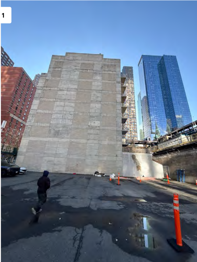
View of West Elevation.
