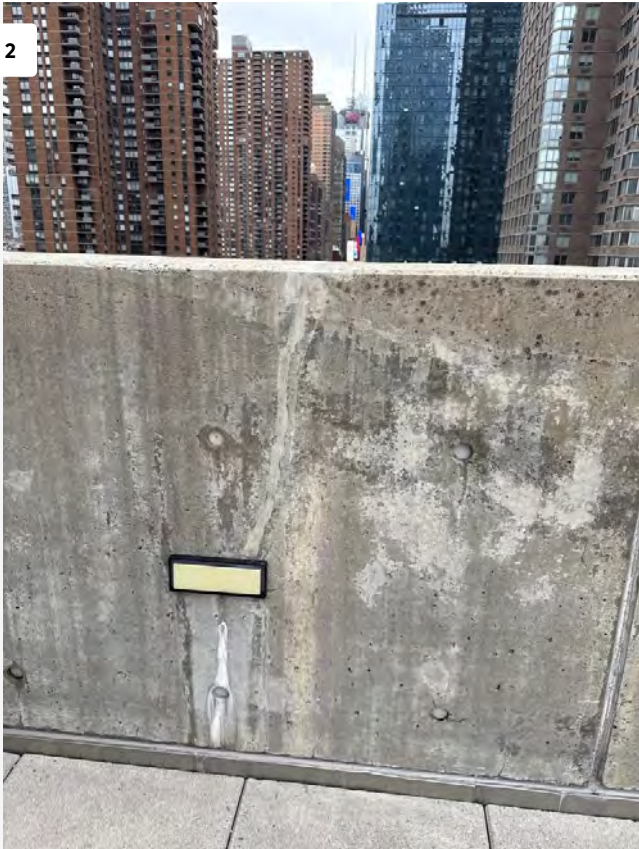
Typical View of Repaired Cracked Concrete at Parapet.
