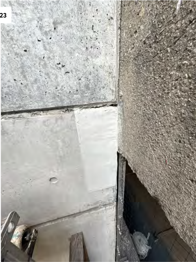
Typical View of Repaired Spalling Concrete at South Elevation.
