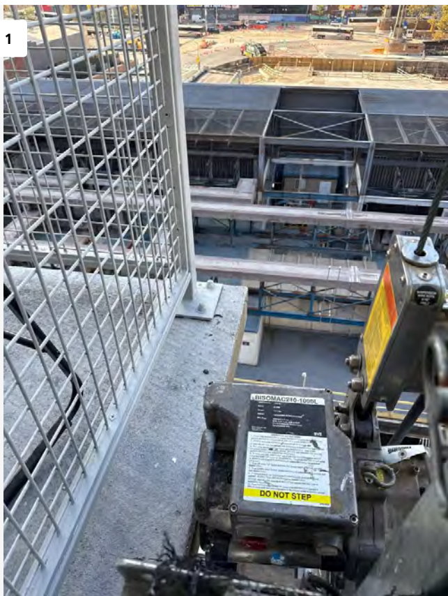
View of QEWI/Close-Up Inspection Conducted during Repair Project.
