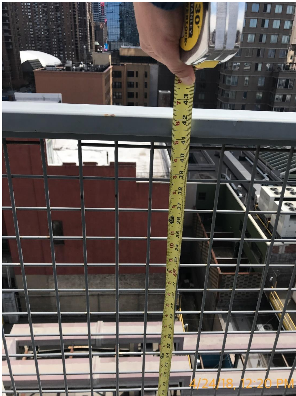
Photo 7. Balcony railing measuring 42 inches in height.
