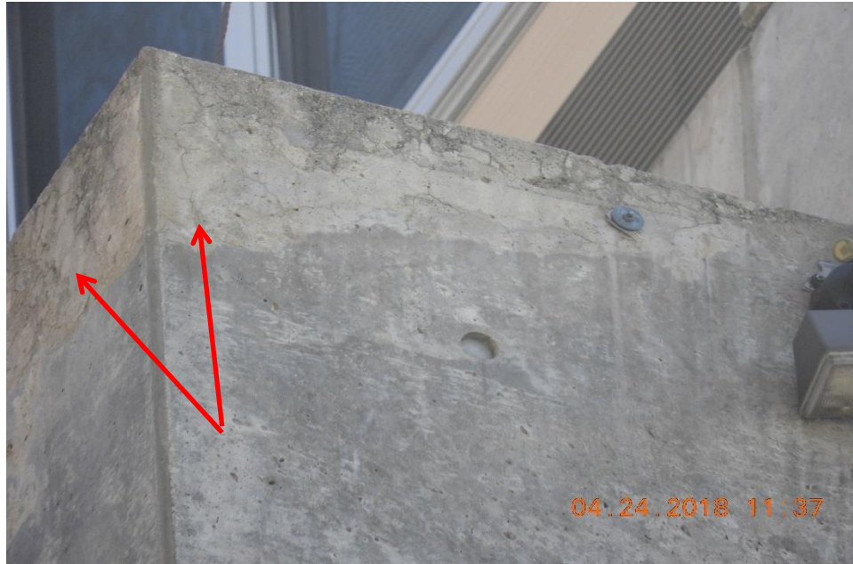
Photo 3. Cracks in setback parapet 8 th floor, north elevation.
