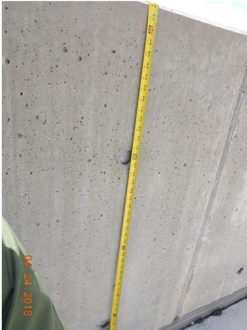
Photo 6. Roof Parapet measuring 50 inches in height.
